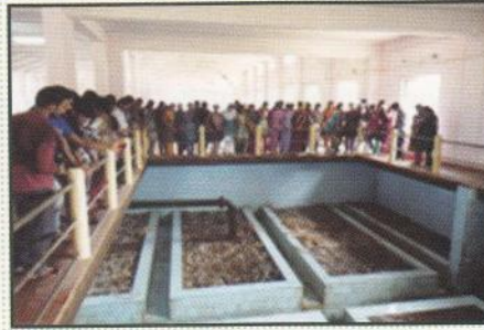
Water Purification Centre Thumbe Mangalore
